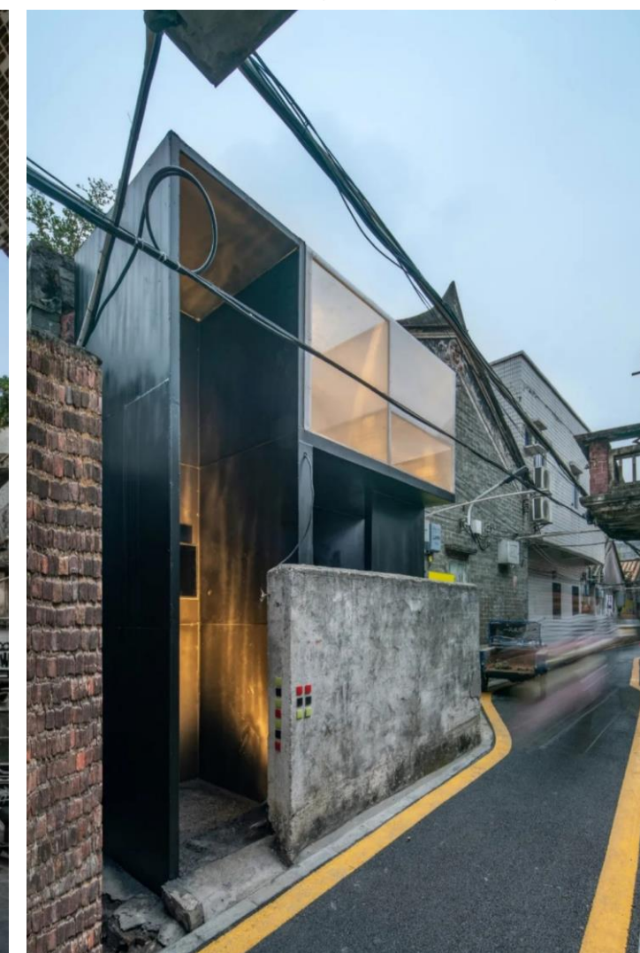
建筑改造后-立方像素空间 Building after reconstruction-Cube Pixel Space
