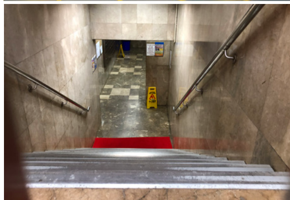
Image 1 Golden Computer Arcade and Golden Building lift lobby on lower ground level
