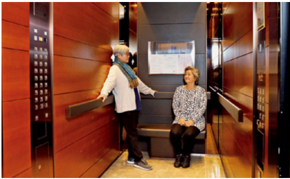
Image 2 Elevators with seats and handrail (Source: HKHS, 2019)
